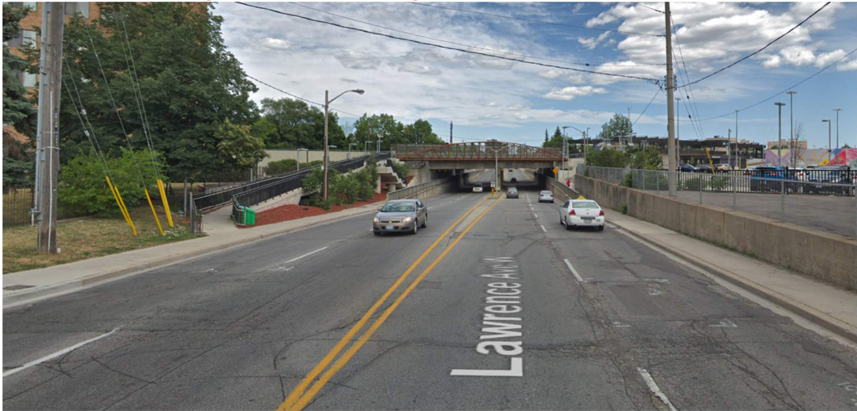
Figure 2-6: Pedestrian Bridge for Direct GO Station Access
