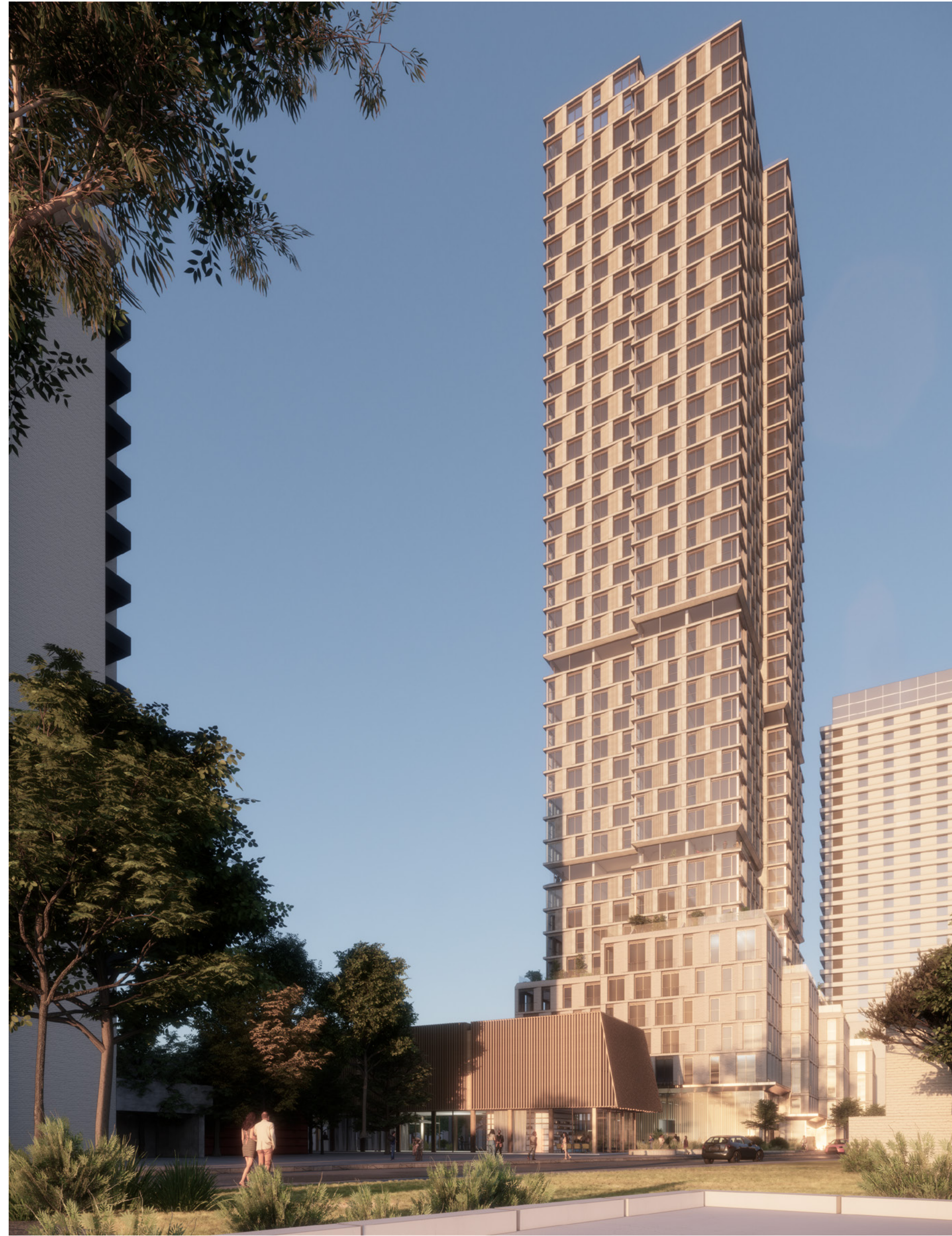
01 - View from East of South Station St.
